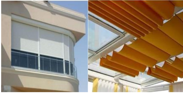
Figure 5. Cover ceilings and windows to reduce heat transfer
