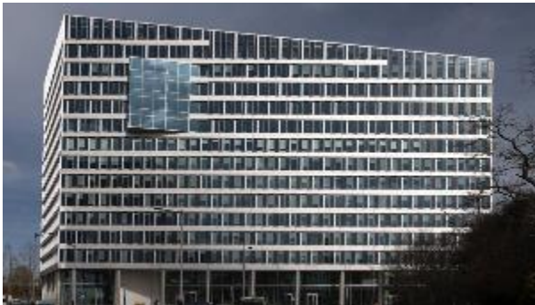
Figure 10 The Edge building
