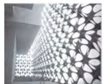
Fig (25)examples for Tiling by means of Plasma –arc cutter
