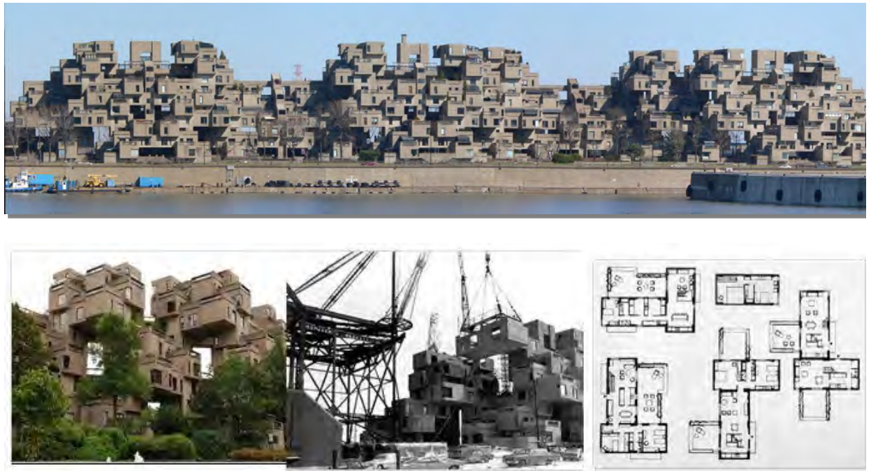
Fig (9) Various views and plans for the 67 project designed by the Israeli Canadian architect Moshe Safdie
