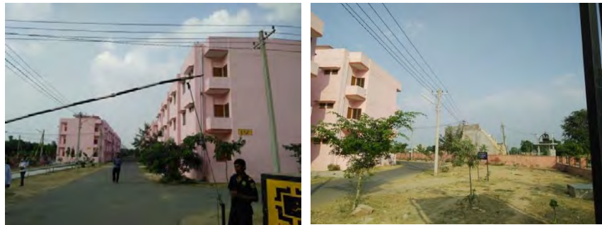
Fig. (11) and (12), BSUP project and the empty piece of land dedicated to the school, Jaisighpura Khor, Delhi Road Jaipur, Rajasthan Source: Photos by the Author
