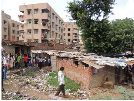
Fig. (23), The in-situ development Vs. the slums, Kailashnagar, Sabarmati in Ahmedabad Source: photo by the author
