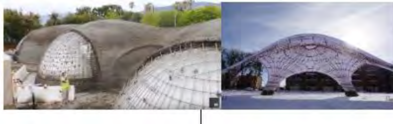
Figure 1. (a) Bini Shells within inflatables covered by a metal mesh as lost reinforcement to be sprayed manually with shotcrete. 1(b) Spray ice on fabric formwork and active bending metallic elements. "Zero bending moment" Lancelot Coar Winnipeg, Canada 2016.
