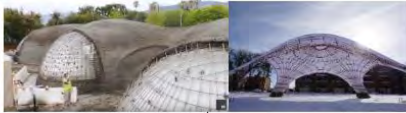
Figure 1. (a) Bini Shells within inflatables covered by a metal mesh as lost reinforcement to be sprayed manually with shotcrete. (b) Spray ice on fabric formwork and active bending metallic elements. "Zero bending moment" Lancelot Coar Winnipeg, Canada 2016.
