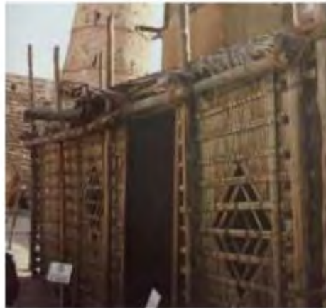
Figure 5. Date Palm Rachis Walls in Arish House (Piesik, 2012)
