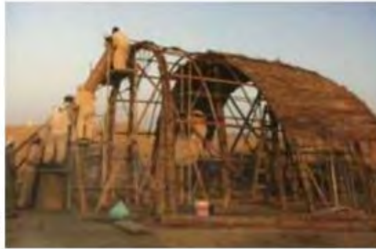
Figure 7. The Vault during Construction (Piesik, 2012)
