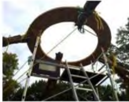
Figure 10. Ring beam in structure (Boisbushet, 2013)
