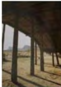
Figure 8. Interior Columns (Piesik, 2012)
