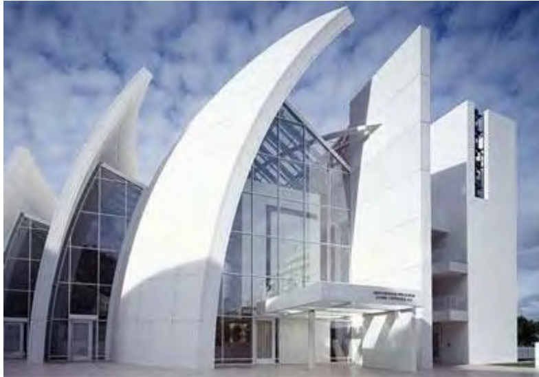
Figure 9. The Jubilee Church built with photo-catalytically active, “self-cleaning”
