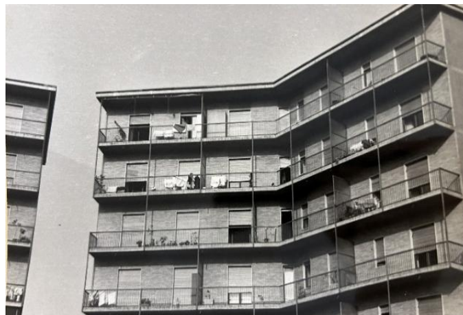
Figure 1. Photo of the inner courtyard taken after construction completion Source. City of Milan, CASVA – Giancesare Battaini Professional Archive.
