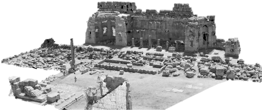
Figure 13. Integrated point cloud model based on TLS and UAV photogrammetry data. (Source: Author, 2025)
