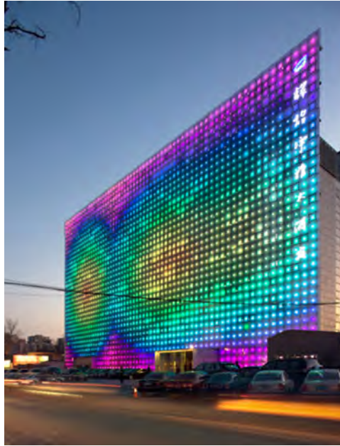
Figure 4. Green pix — Zero Energy Media Wall-, Beijing source: www.archdaily.com
