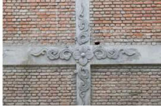
Figure 11 Example of decorative concrete cast
