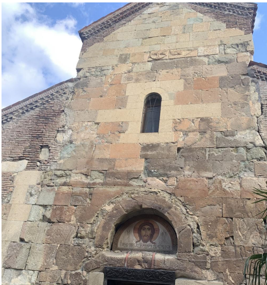
Figure 1. Anchiskhati Basilica - main entrance. Note. Photograph by N. Dzebisashvili, 2025.
