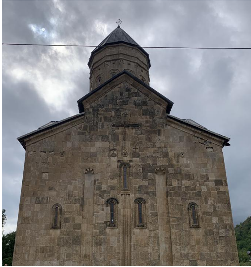
Figure 3. Barakoni Church - eastern facade. Note. Photograph by N. Dzebisashvili, 2025.
