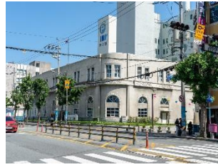
Figure 15. U.S. Embassy and U.S. Information Service, No. 10 of Figure 16. Source. Busan Metropolitan City (2019)
