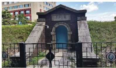
Figure 9. The Bokbyeongsan Mt. Drainage area, No. 4 of Figure 16. Source. Busan Metropolitan City (2025a)
