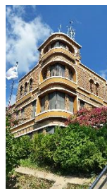
Figure 7. The National Central Observatory No. 3 of Figure 16. Source. Busan Metropolitan City (2019)
