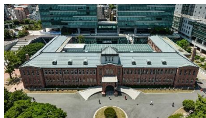
Figure 12. Temporary Government Complex, No. 6 of Figure 16. Source. Busan Metropolitan City (2019)
