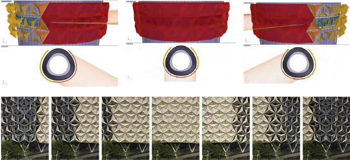
Figure 13. The Kinetic process of the shading system which track the sun location
