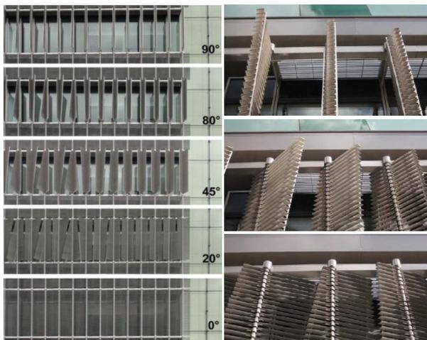
Figure 10. Different states of the sun-shading kinetic system
